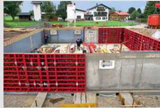
Wall Formwork
